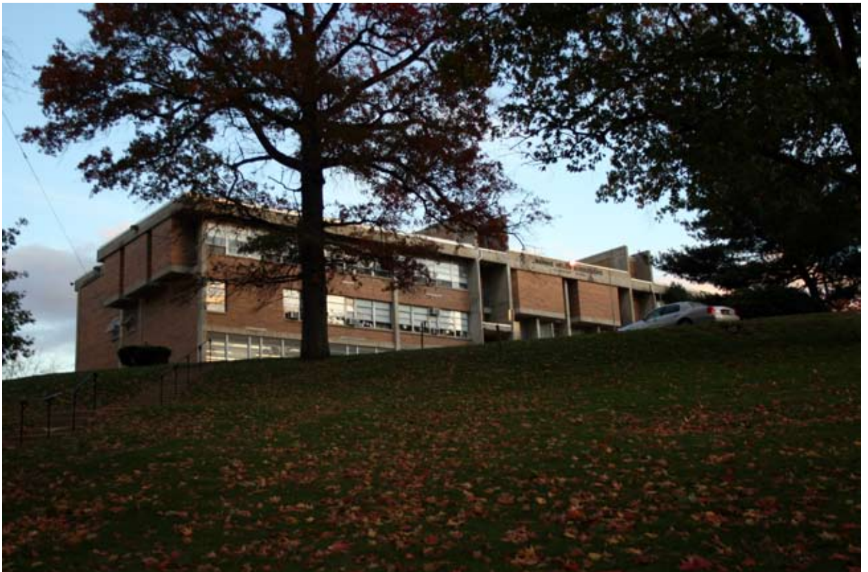
(below) The 1971 elementary school building
