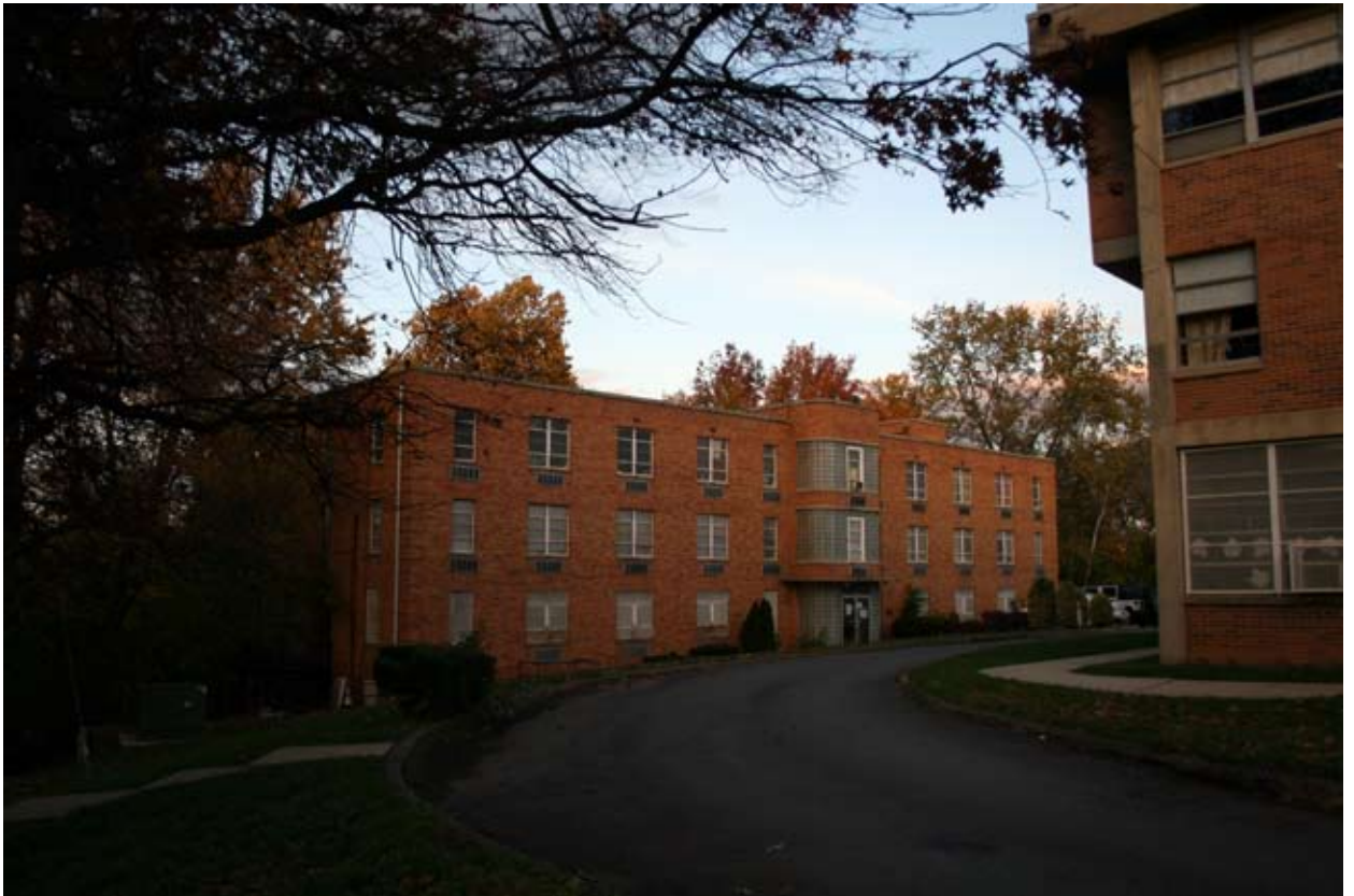
Image 55 (above) the 1956 dormitory as it currently stands, used as a community center by the District of Columbia
