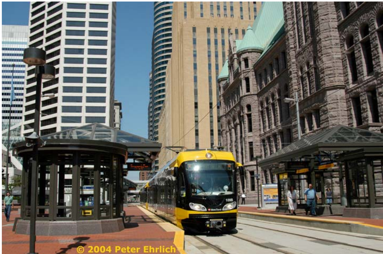
Figure 6: Light rail car at the Government Plaza Station. Notice how the station's design complements that of the Municipal Building (which serves as the Minneapolis City Hall and the Hennepin County Seat), demonstrating that transit stops linked to neighborhood identity have spread beyond Lowertown.
